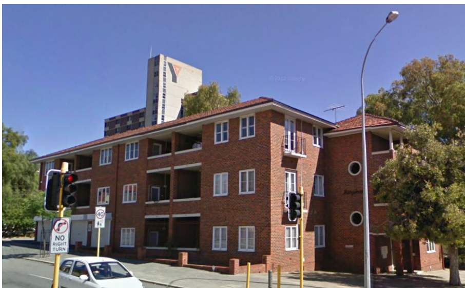
Marginata Flats on the north-west corner of Goderich and Hill Streets in Perth (Google 2013).
